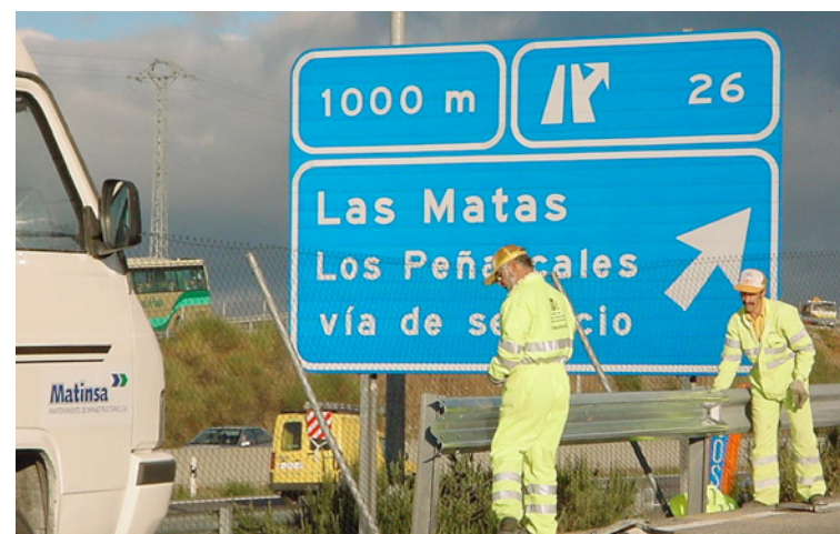
Installing a metal barrier
