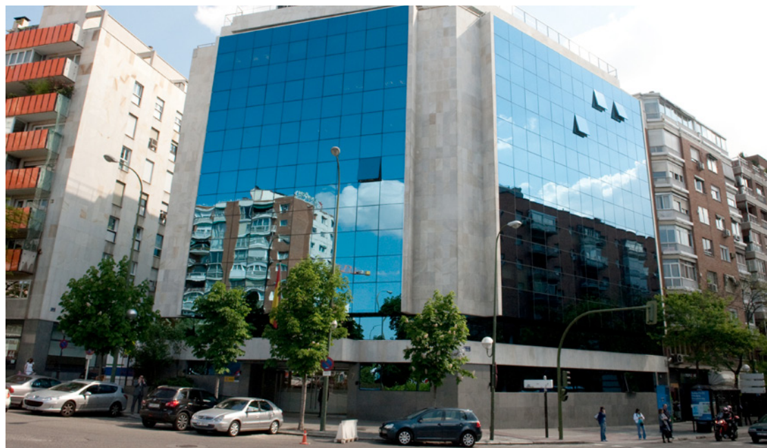
Road Infrastructure's General Direction headquarters rehabilitation, Madrid
