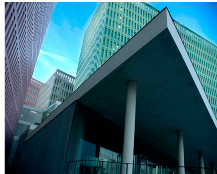
City of Justice complex in Barcelona
